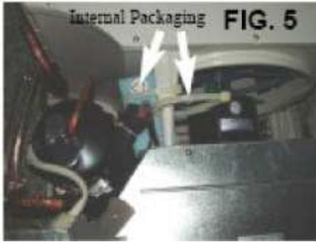
10. Your unit may come with internal packaging. These packaging materials must be removed before re-inserting the air conditioner back into cabinet. Fig. 5.
